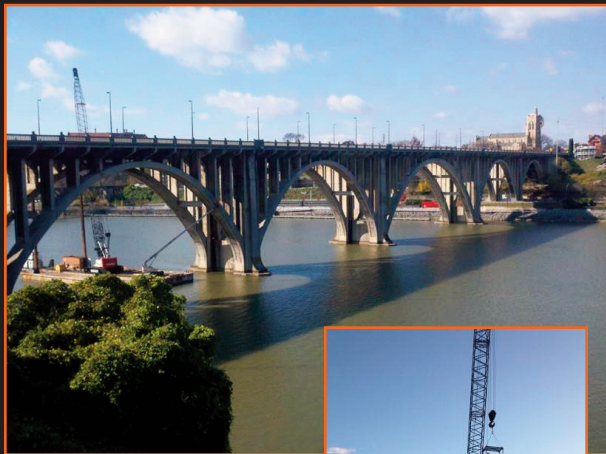
Henley Street Bridge
